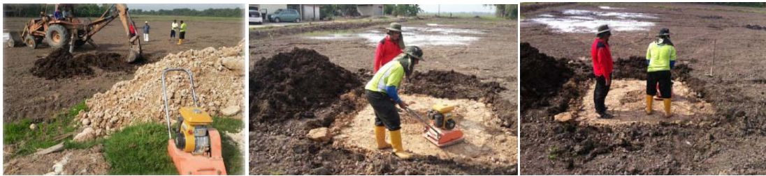
Replacement of submerged soil
