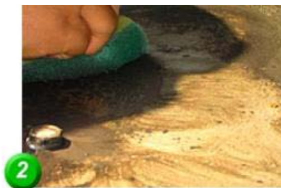
Application of industrial degreaser with a normal sponge.
