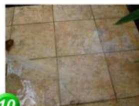
10 The floor is thoroughly cleaned from oil.
